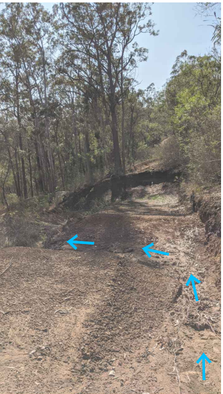
PHOTO 8: GOOD EXAMPLE OF INCORPORATING WATER TURN OUTS INTO TRAIL DESIGN.
