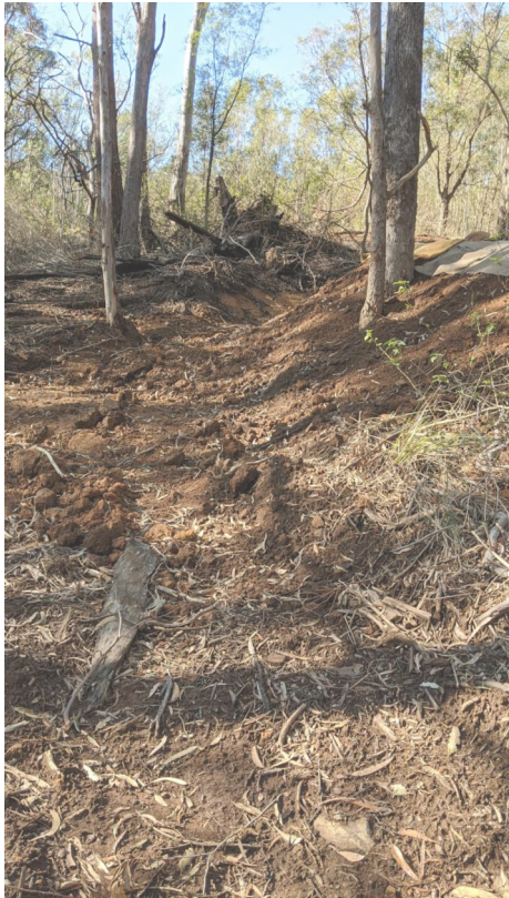
PHOTO 3: STABILISE DOWNSLOPE SIDE OF ALL BATTERS/BERMS WITH LEAF LITTER/MULCH OR JUTE MATTING. TYPICAL FOR ALL BATTERS/BERMS. REFER TO DETAIL 1 ON ESCP04.
