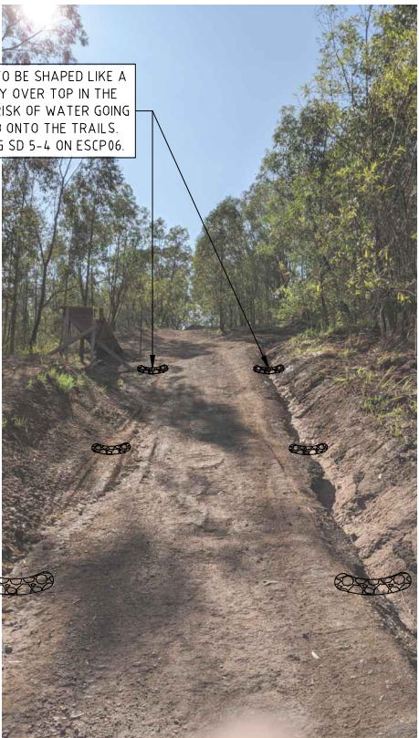
PHOTO 7: NOTE CONCENTRATED FLOWS RUNNING DOWN EITHER SIDE OF ACCESS TRAIL CAUSING RILLING. RESHAPE AND PROVIDE ROCK 'CHECK' DAMS TO MINIMISE RUNOFF VELOCITIES. WHERE POSSIBLE TURN WATER OUT OFF TRAIL. REFER TO DETAILS 7 ON ESCP05 AND PHOTO 11.
