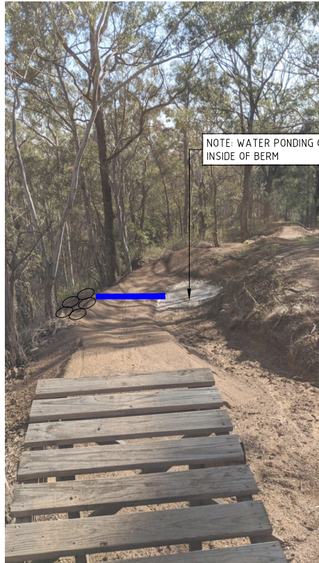
PHOTO 1: PROVIDE RELIEF CULVERT UNDER BERM TO MINIMISE RISK OF WATER PONDING ON TRAIL. PROVIDE ROCK RIP RAP AT OUTLET TO MINIMISE RISK OF SCOURING.
