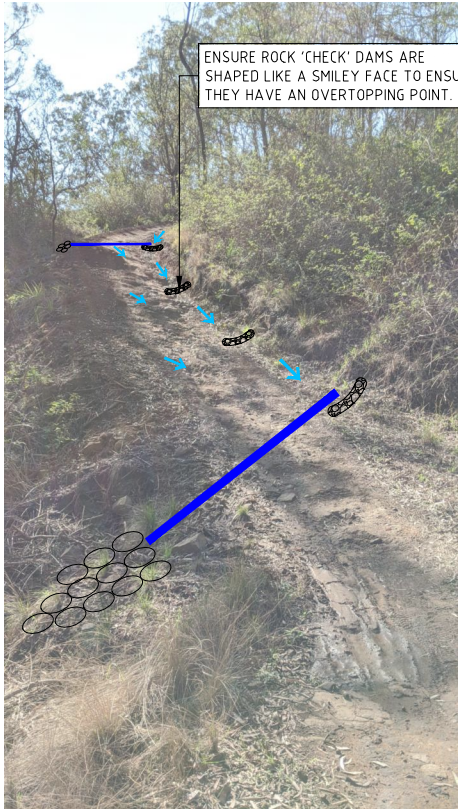
PHOTO 2: PROVIDE ROCK 'CHECK' DAMS AND RELIEF CULVERTS OR GRAVEL DRAINS (REFER TO DETAILS 4 & 6 ON ESCP04 AND STANDARD DRAWING SD 5-4 ON ESCP06) UNDER TRAIL TO DISPERSE WATER AT REGULAR INTERVALS. PROVIDE ROCK RIP RAP AT CULVERT/DRAIN OUTLETS TO MINIMISE RISK OF SCOURING.
