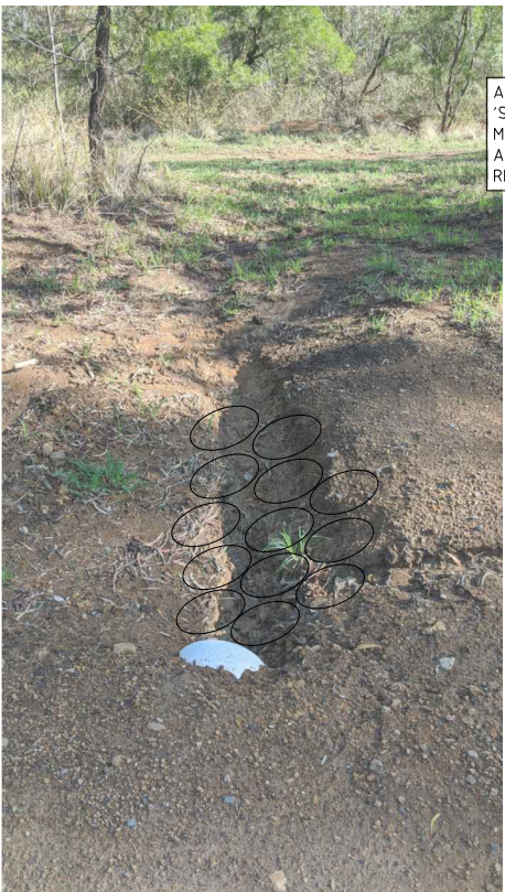
PHOTO 6: NOTE EROSION AT OUTLET OF RELIEF CULVERT. RESHAPE DISH DRAIN AND PROVIDE ROCK RIP RAP AT OUTLET OF ALL RELIEF CULVERTS TO MINIMISE RISK OF FURTHER EROSION. REFER TO DETAIL 4.
