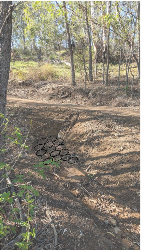
PHOTO 4: GOOD USE OF RELIEF CULVERT. HOWEVER, PROVIDE ROCK RIP RAP AT OUTLET OF ALL RELIEF CULVERTS TO MINIMISE RISK OF FURTHER EROSION. REFER TO DETAIL 4.
