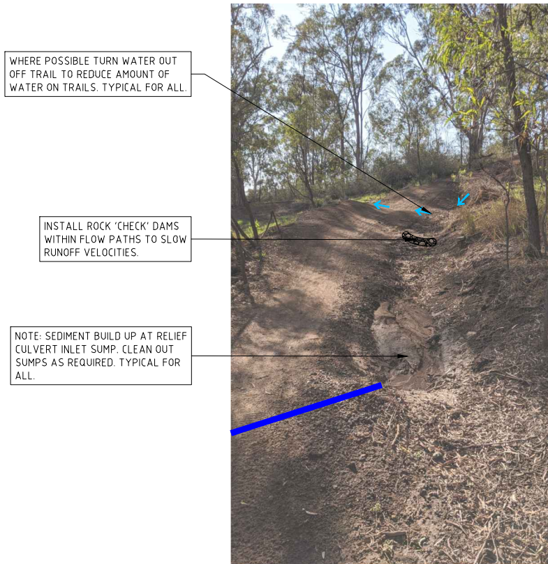
PHOTO 5: REMOVE BUILD UP OF SEDIMENT AT RELIEF CULVERT INLETS AS REQUIRED. REFER TO DETAIL 4.
